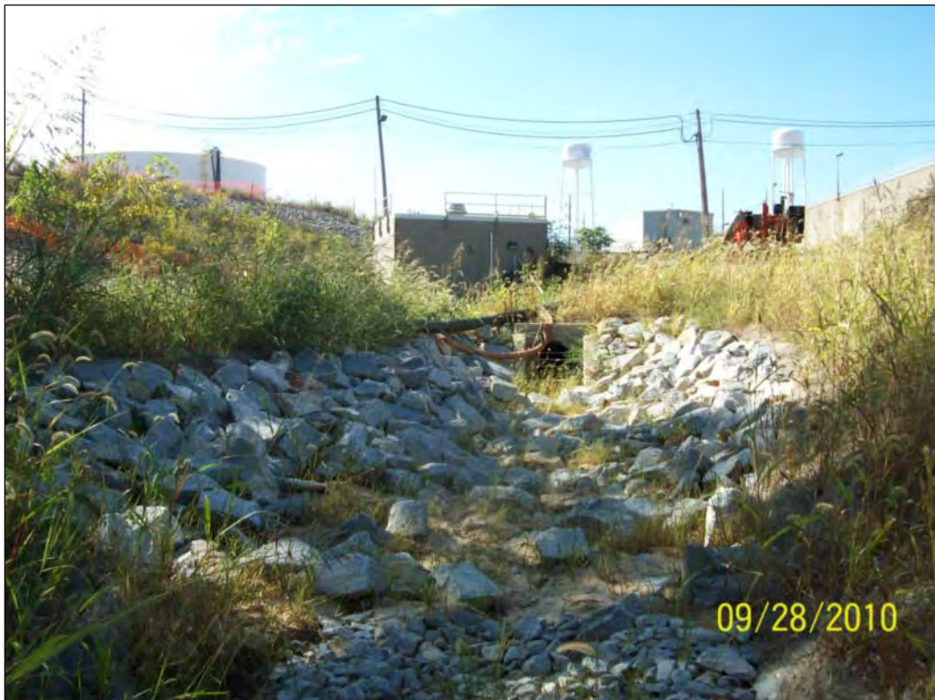
FIGURE 2.0 - PARCEL 3, LOCATION 2, LOOKING UPSTREAM (WEST)
