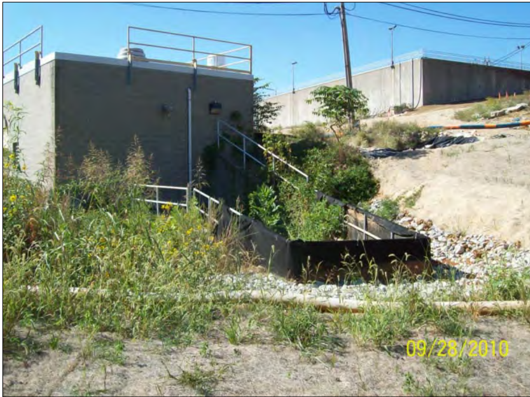
FIGURE 1.0 - PARCEL 3, LOCATION 1, LOOKING UPSTREAM (WEST)
