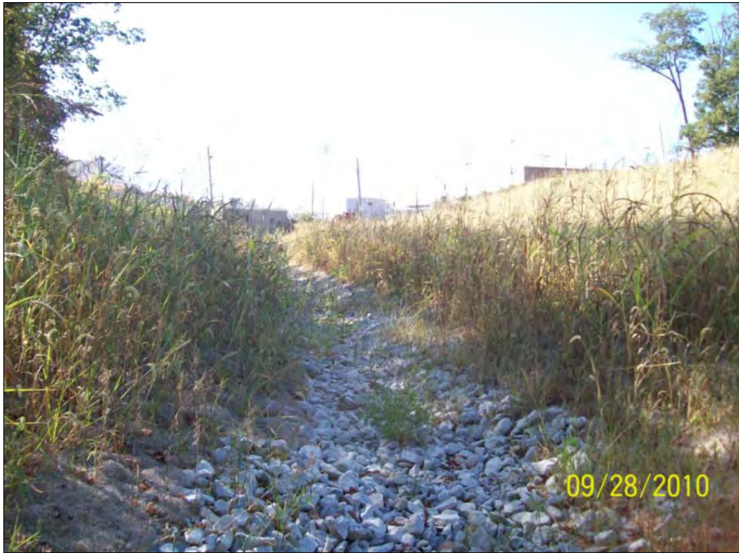
FIGURE 3.0 - PARCEL 3, LOCATION 3, LOOKING UPSTREAM (WEST)
