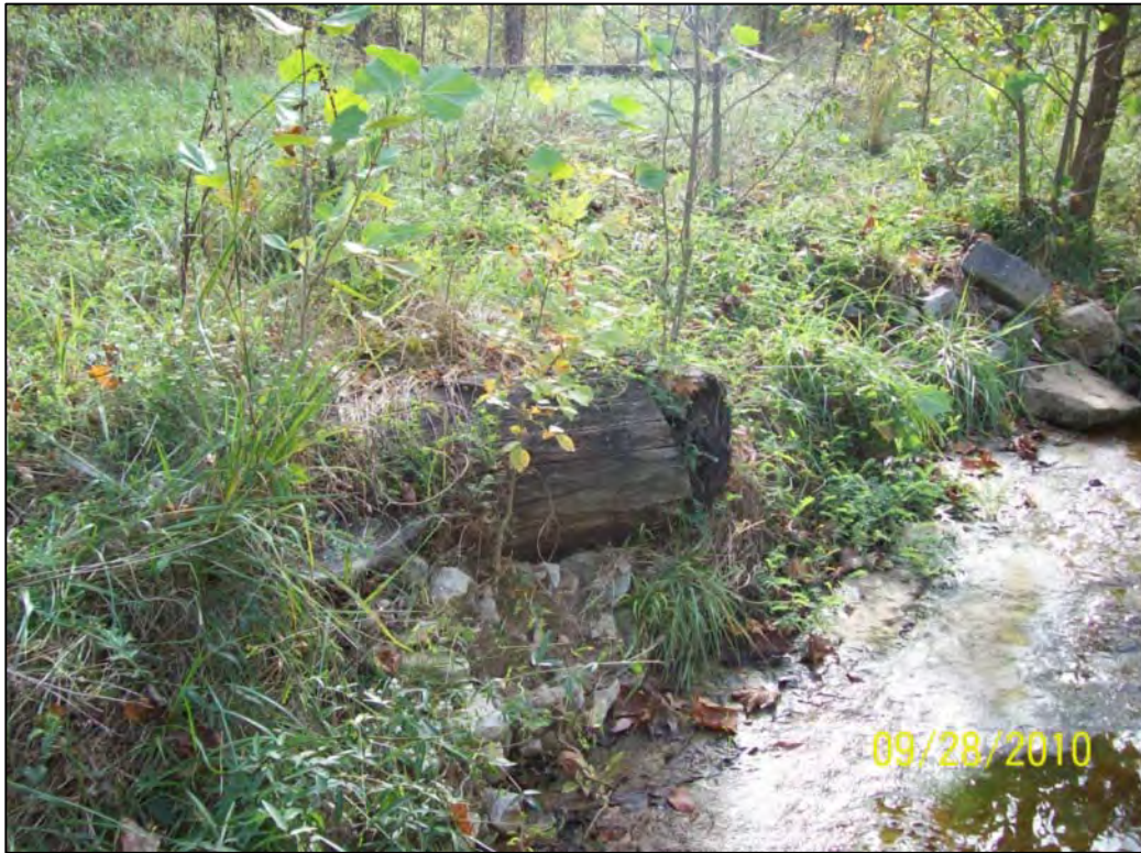
FIGURE 7.4 - PARCEL 6, LOCATION 7, LOG DEFLECTOR
