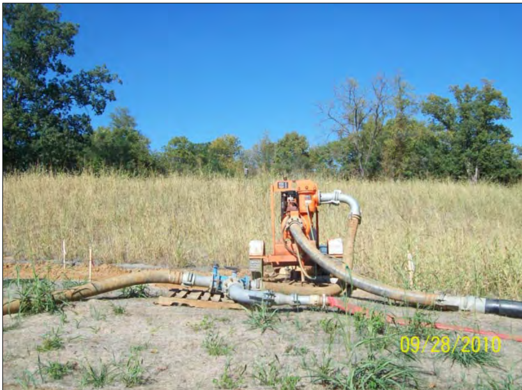
FIGURE 1.3 - PARCEL 3, LOCATION 1, LOOKING NORTH, RIGHT BANK
