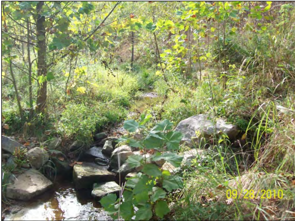
FIGURE 7.0 - PARCEL 6, LOCATION 7, LOOKING UPSTREAM (ROCK WEIR)
