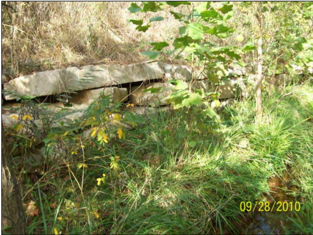
FIGURE 6.2 - PARCEL 6, LOCATION 6, LOOKING DOWNSTREAM ROUGHBACK WALL (STABLE - NO MOVEMENT)
