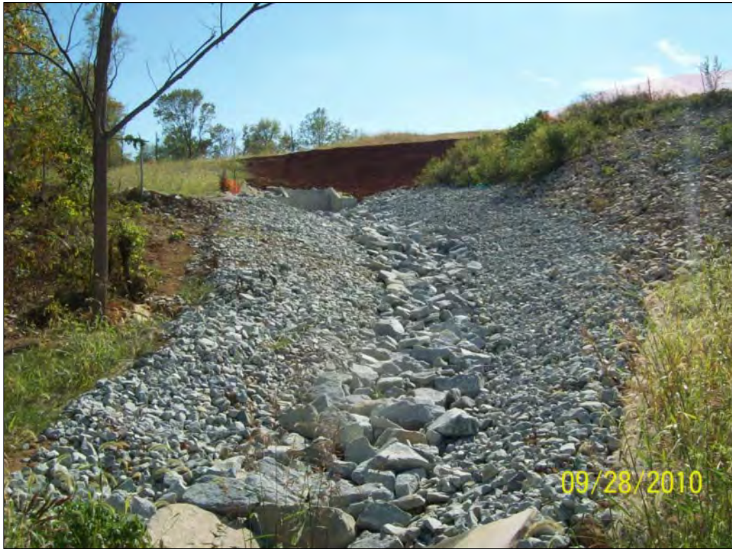
FIGURE 1.2 - PARCEL 3, LOCATION 1, LOOKING SOUTH, TRIBUTARY FROM PARCEL 201
