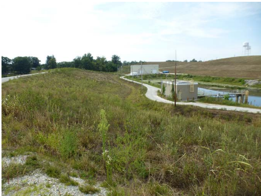
PP11 Area 5 View South, September 5, 2013
