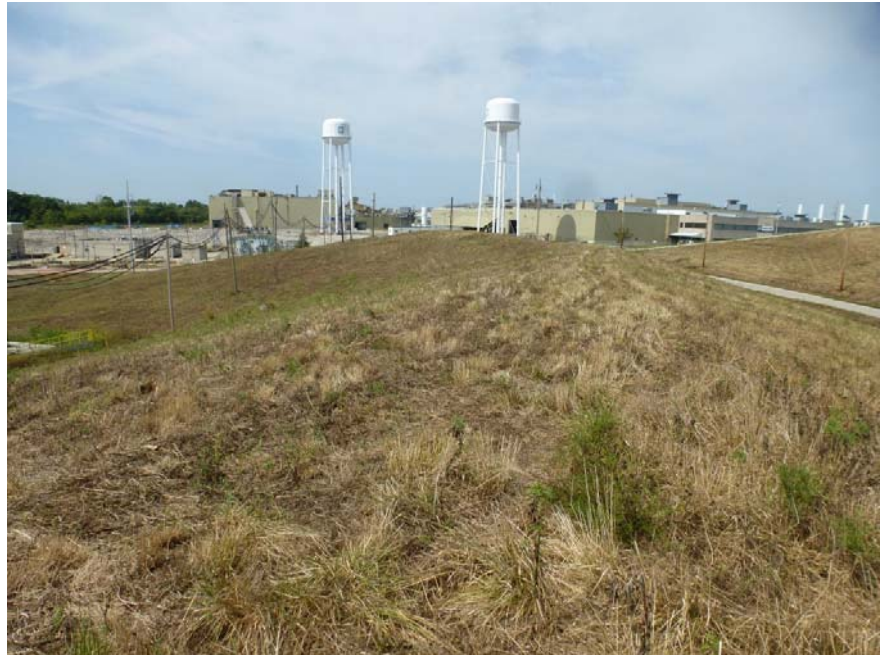
PP 6 Area 2 View West, September 5, 2013
