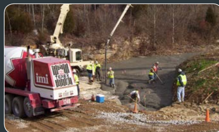
CONCRETE WORK IN THE SPRING 018 AREA
