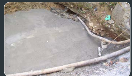
SPRING 018 COLLECTION BERM REINFORCEMENT
