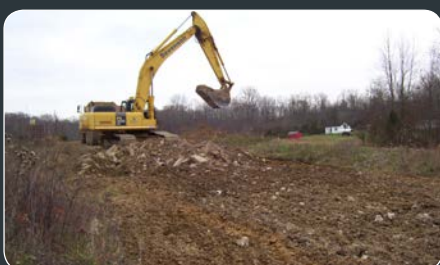
HAUL ROAD REMOVAL WEST OF PEERLESS ROAD
