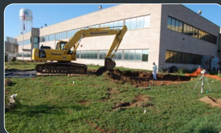
ADDITIONAL EXCAVATION IN FRONT LAWN OF WEST PLANT AREA
