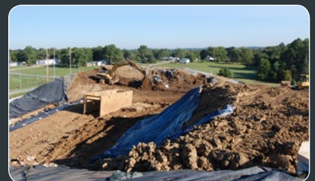
EAST PLANT AREA FINAL COVER SYSTEM GRADING ACTIVITIES
