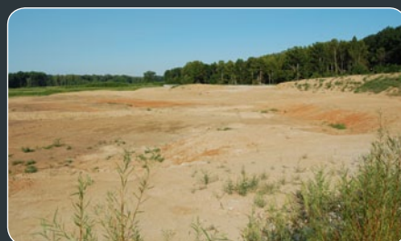
COMPLETED EXCAVATION WEST OF PEERLESS ROAD
