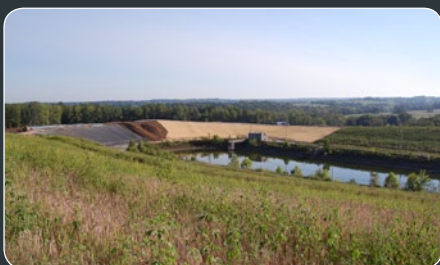
EAST PLANT AREA COVER SYSTEM PROGRESS NORTH OF STORM WATER POND
