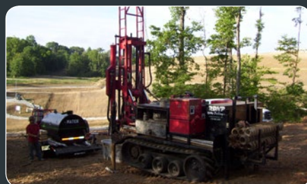
DRILLING ACTIVITIES ALONG PROPOSED TRENCH ALIGNMENT
