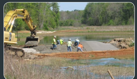
REPAIRING THE POND OVERFLOW STRUCTURE NORTH OF BROOMSAGE ROAD
